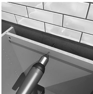
Drill a pilot hole (same size as your masonry bit) through the cross brace, then, with your 200 mm drill bit, drill directly into the wall behind and inset your wall plug
