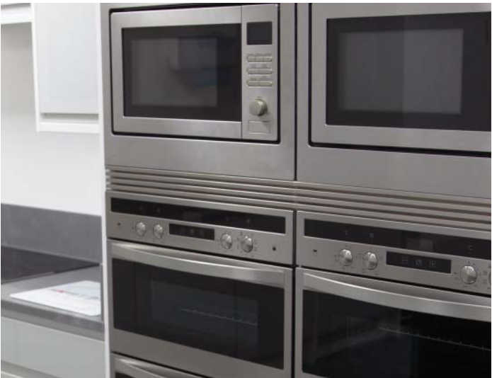
Photo shows use of two grills, cut to reduced height
